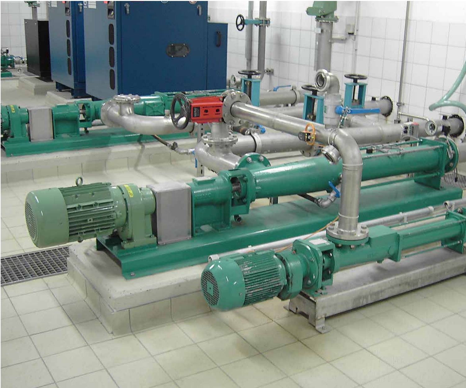
NEMO® progressing cavity pumps convey digested sludge
